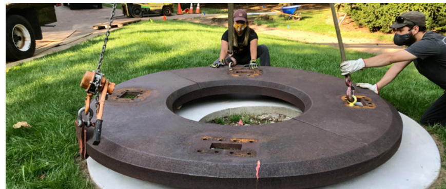
[ Top Left Photo: Before, uncovering old hardware that had deteriorated over time on Split Ritual II ; Top Right: Before, interior view of peeling/lifting paint on Untitled ; Bottom: After, setting the base on the new foundation on Split Ritual ]
