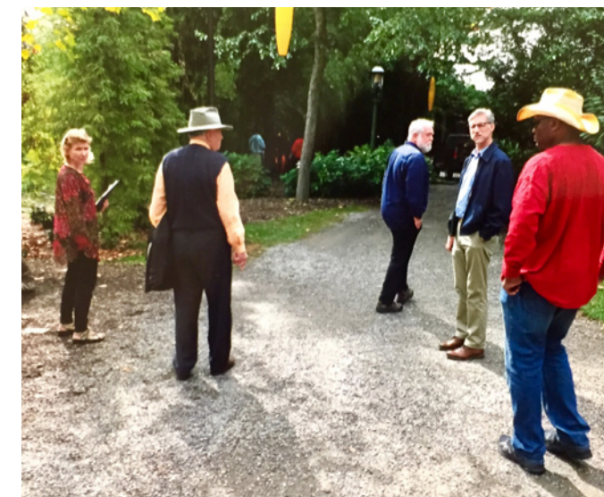
Top Photo: With Michael Unger and Brian Carey at construction site of the Seward Johnson Center for the Arts building; Bottom: Site planning for new installation with Claire Brown, Charles Haude, Michael Unger, and Autin Wright
