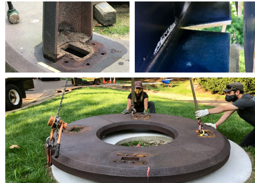
Top Left Photo: Before, uncovering old hardware that had deteriorated over time on Split Ritual II ; Top Right: Before, interior view of peeling/lifting paint on Untitled ; Bottom: After, setting the base on the new foundation on Split Ritual II
